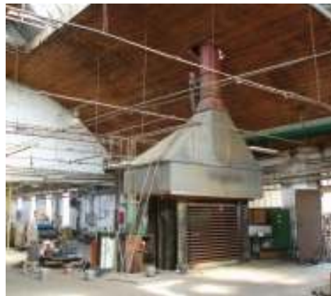
Complete repair of press for plywood production
