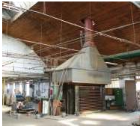
Complete repair of press for plywood production
